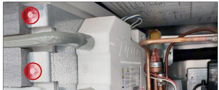
Fig. 3. TrueZone UV system side view. TrueZone bracket screw locations.
