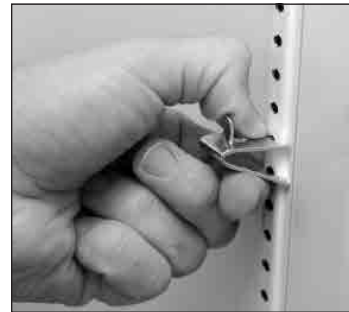
Fig. 3. You may need to squeeze or twist the bottom of the shelf clip to install.
