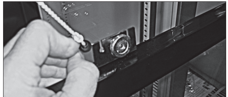
Fig. 8. Slide the black tab holding the door cord out the roller bracket's back.
