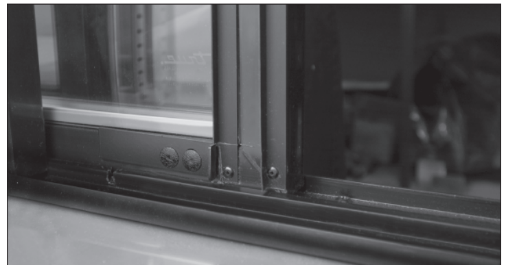
Fig. 2. Door latch is in the closed position (disengaged from notch).
