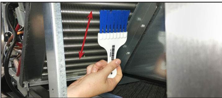
Fig. 3. Never brush across the coil fins.
