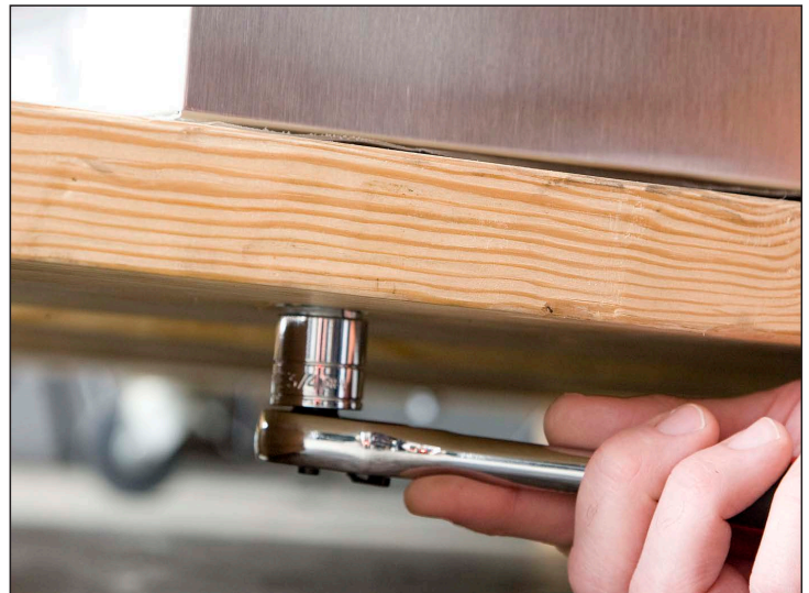
Fig. 3. Remove the skid bolts.
