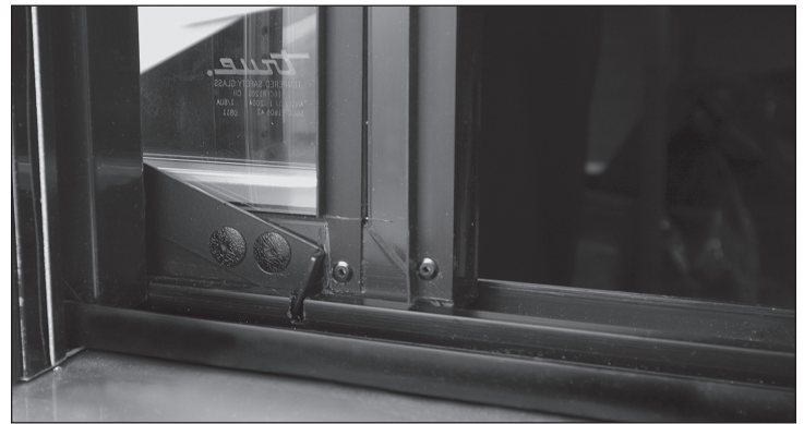
Fig. 1. Door latch is in the open position (engaged with notch).
